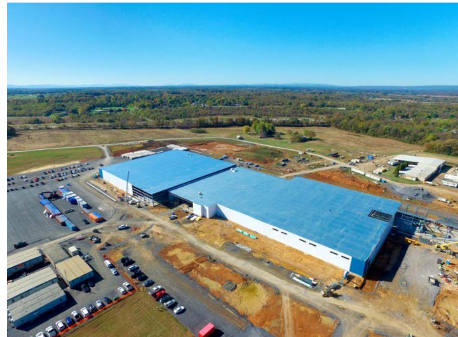
→ Solid progress: New factory in Ranson, West Virginia
